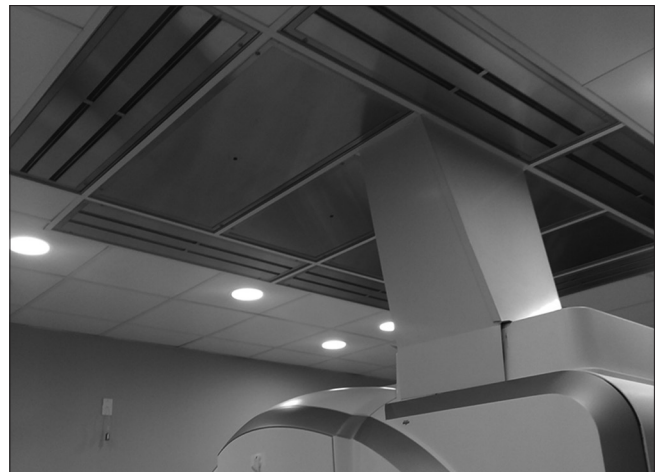
Figure 4: View of the air flow system demonstrating the air curtain outlets surrounding the laminar flow diffusers.
